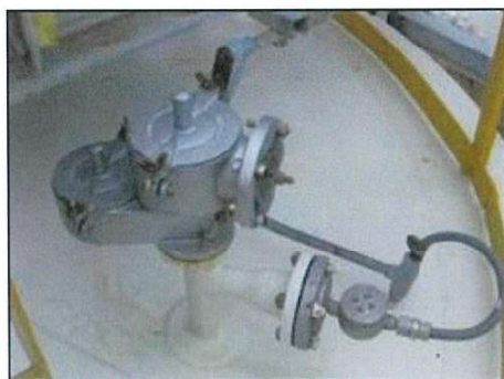
Pressure Vacuum Relief Valve
